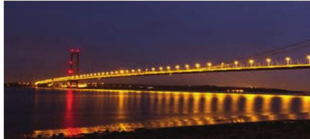
Source: www.nelps.wordpress.com Picture 11.1 Humber Bridge
