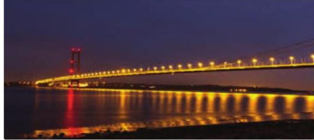
Source: www.nelps.wordpress.com Picture 11.1 Humber Bridge
